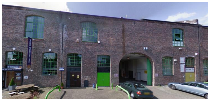
Then followed the Century Buildings in Brunswick Business Park
